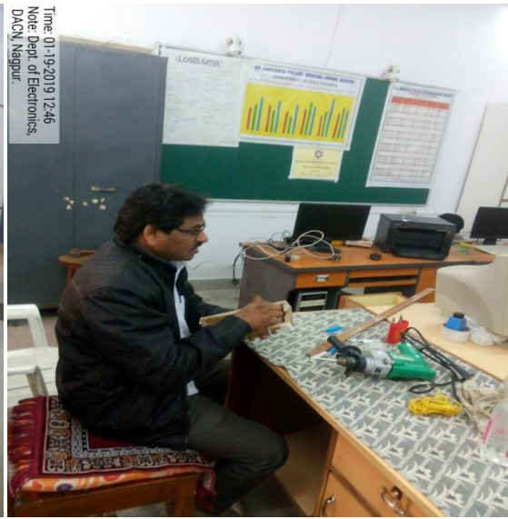
Shri Ram Ghode installing the Electrical board
