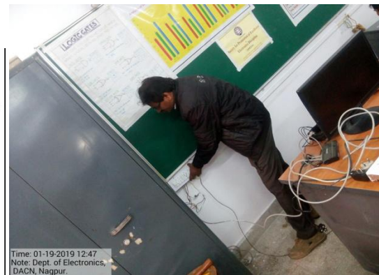
Shri Ram Ghode doing Electrical work
